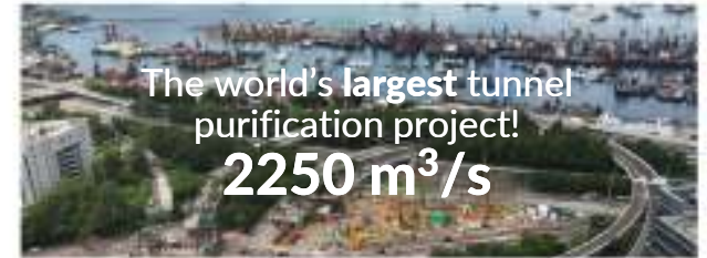
2021: CENTRAL KOWLOON TUNNEL, HONG KONG 9 APS stations, with an air purification volume of 2,250 m 3 /s
