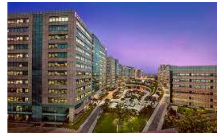
AHU Purification Project, India
