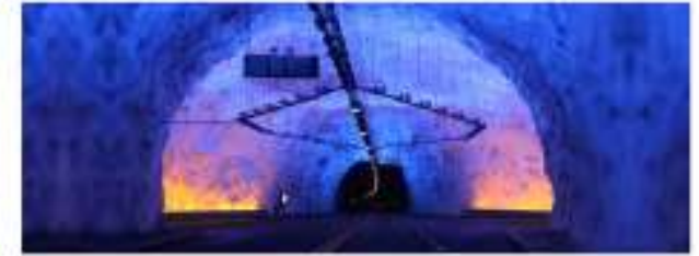
2001: LAERDAL TUNNEL The world's longest tunnel equipped with Air Purification System, 24.5 KM
