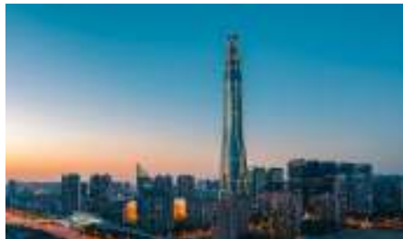
Tianjin CTF Finance Center
